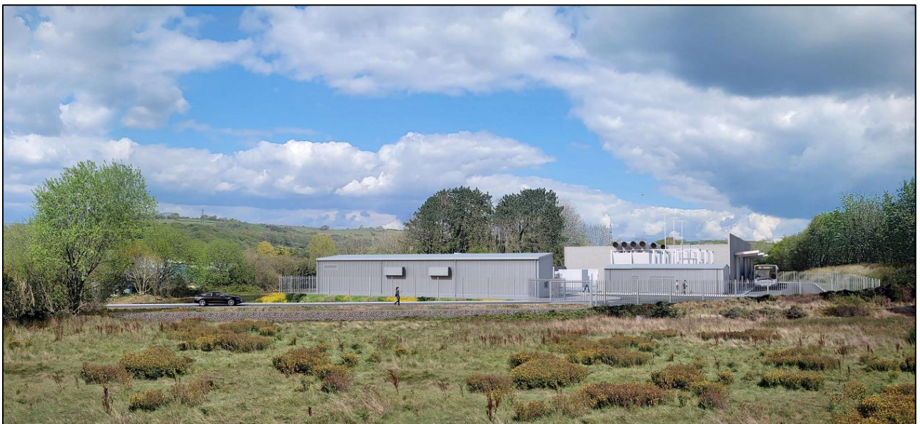
Figure 3: Eye Level View of Hydrogen Production Facility from West of Site
