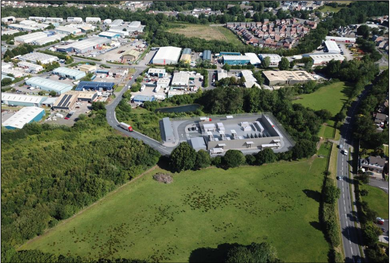
Figure 2: Birds Eye View of Hydrogen Production Facility inc.8 m High Wall and Immediate Surroundings
